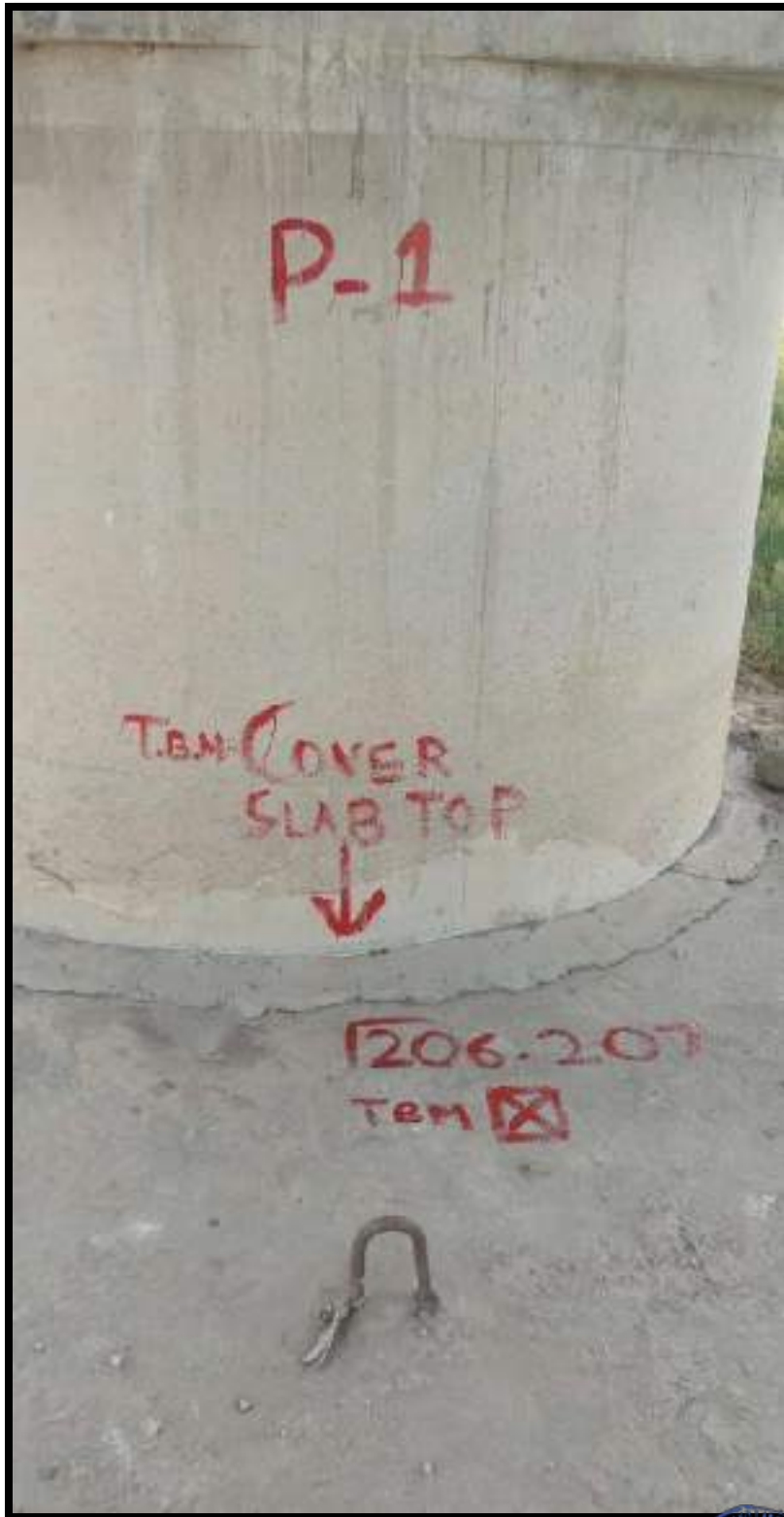
PHOTOGRAPH 12: Photograph showing elevation of the Benchmark of Kotbudha/Bandala River Bridge.
