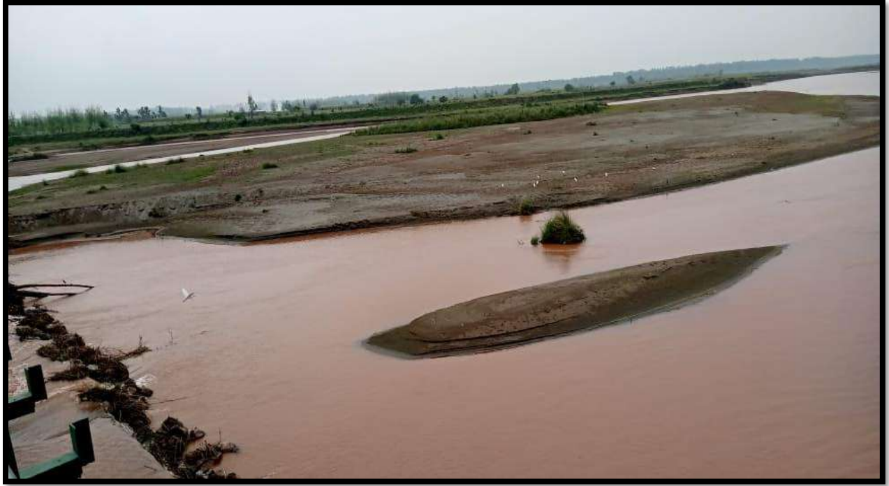
PHOTOGRAPH 7: Desilting sand zone in Ravi River, Gurdaspur district.
