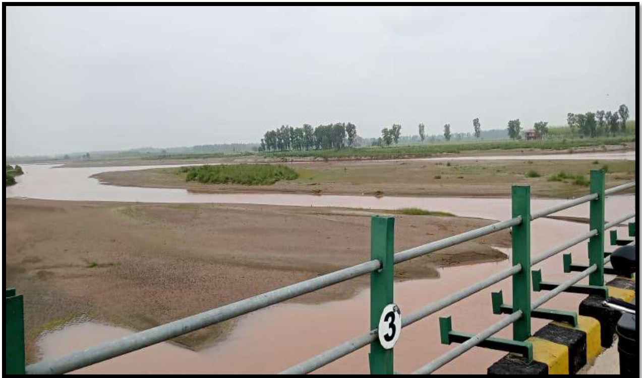
PHOTOGRAPH 8: Desilting sand zone in Ravi River, Gurdaspur district.
