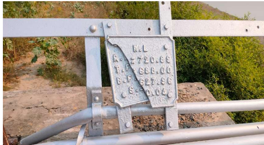
Mandi Kalu Railway Bridge
